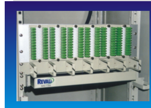
VISTA FRONTAL DO STOV-4300 144 FIBRAS COM ADAPTADORES, PAINEL GUIA E SAC-1300
